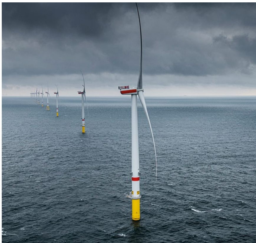
BKR2 has an operating capacity of approximately 465 MW and is located 59km off the coast of Lower Saxony in the North Sea, Germany.
