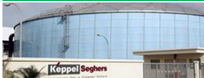
Keppel Seghers Ulu Pandan NEWater Plant
