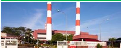
Senoko WTE Plant
