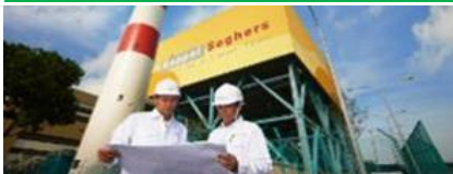
Keppel Seghers Tuas WTE Plant
