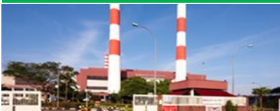
Senoko WTE Plant
