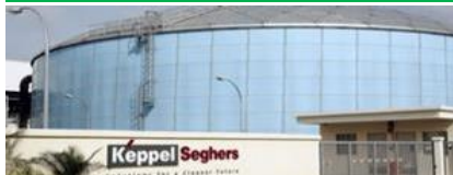
Keppel Seghers Ulu Pandan NEWater Plant
