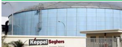
Keppel Seghers Ulu Pandan NEWater Plant
