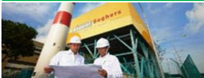
Keppel Seghers Tuas WTE Plant
