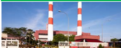
Senoko WTE Plant
