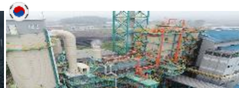
EMKH – Integrated Waste Platform 1
