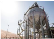
Aramco Gas Pipelines Company
