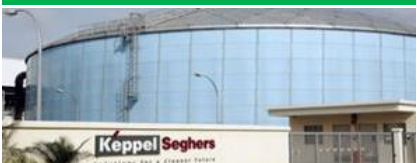
Keppel Seghers Ulu Pandan NEWater Plant
