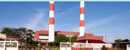
Senoko WTE Plant
