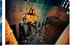
Keppel Seghers Tuas WTE Plant
