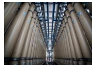
Keppel Seghers Ulu Pandan NEWater Plant
